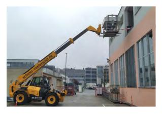
The first dimensional stability furnace is carefully lifted out of the building opening
