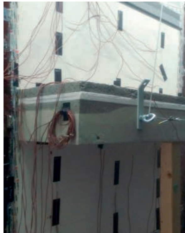
† Mounting an exterior wall construction with concrete ceiling in the test stand to investigate thermal bridge effects in interior insulation
