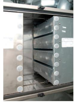
Purification filters for intake-air
